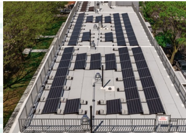
Repaired roof and solar panel system at Berry St Houses
