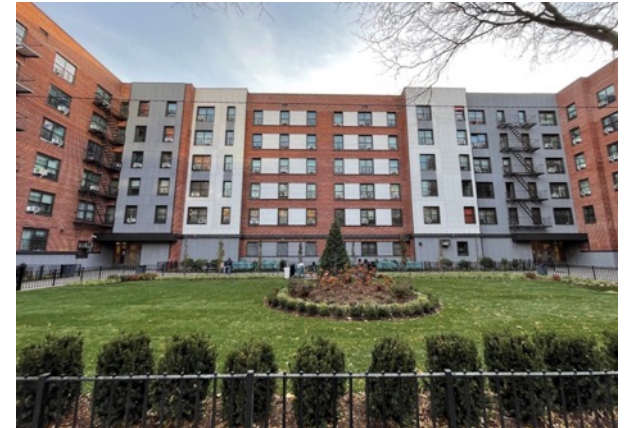
Site improvements at Warren St Houses
